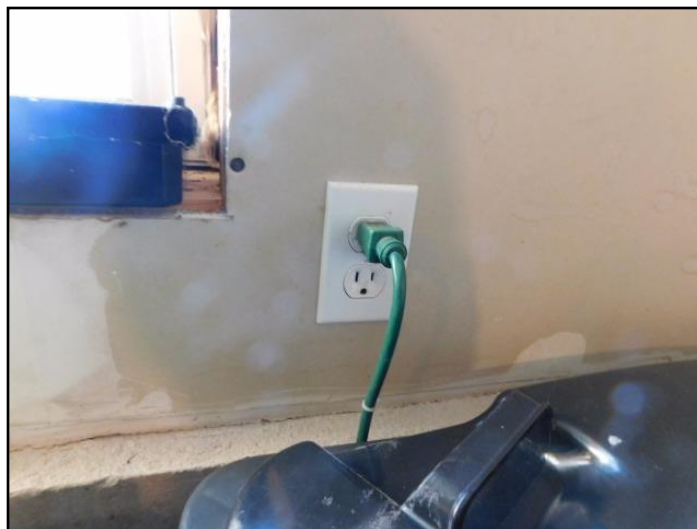
12. No GFCI/GFI (Ground Fault Circuit...
