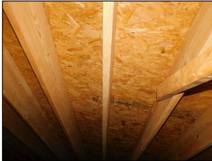
7. Oriented Strand Board (OSB) sheathing
