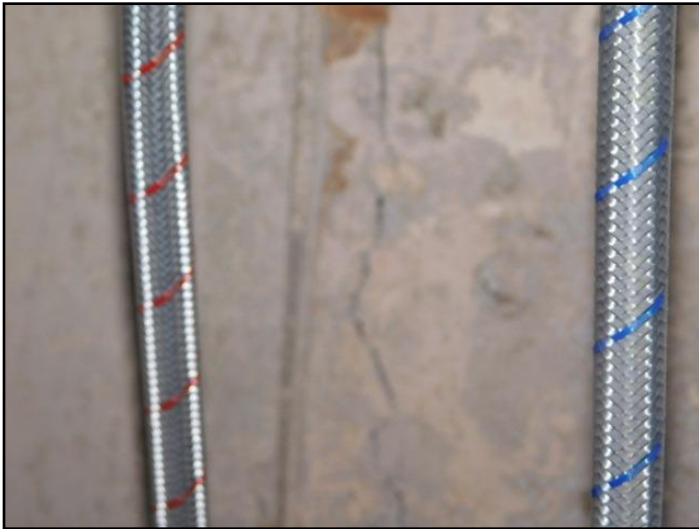
8. Typical minor cracks
