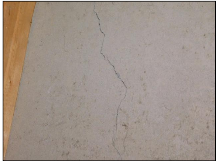
9. Typical minor cracks
