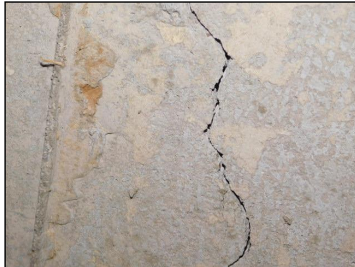
10. Typical minor cracks
